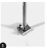
Fix clips with suitable screws (min. 2 per metre/40"). Drill cable holes if required.
